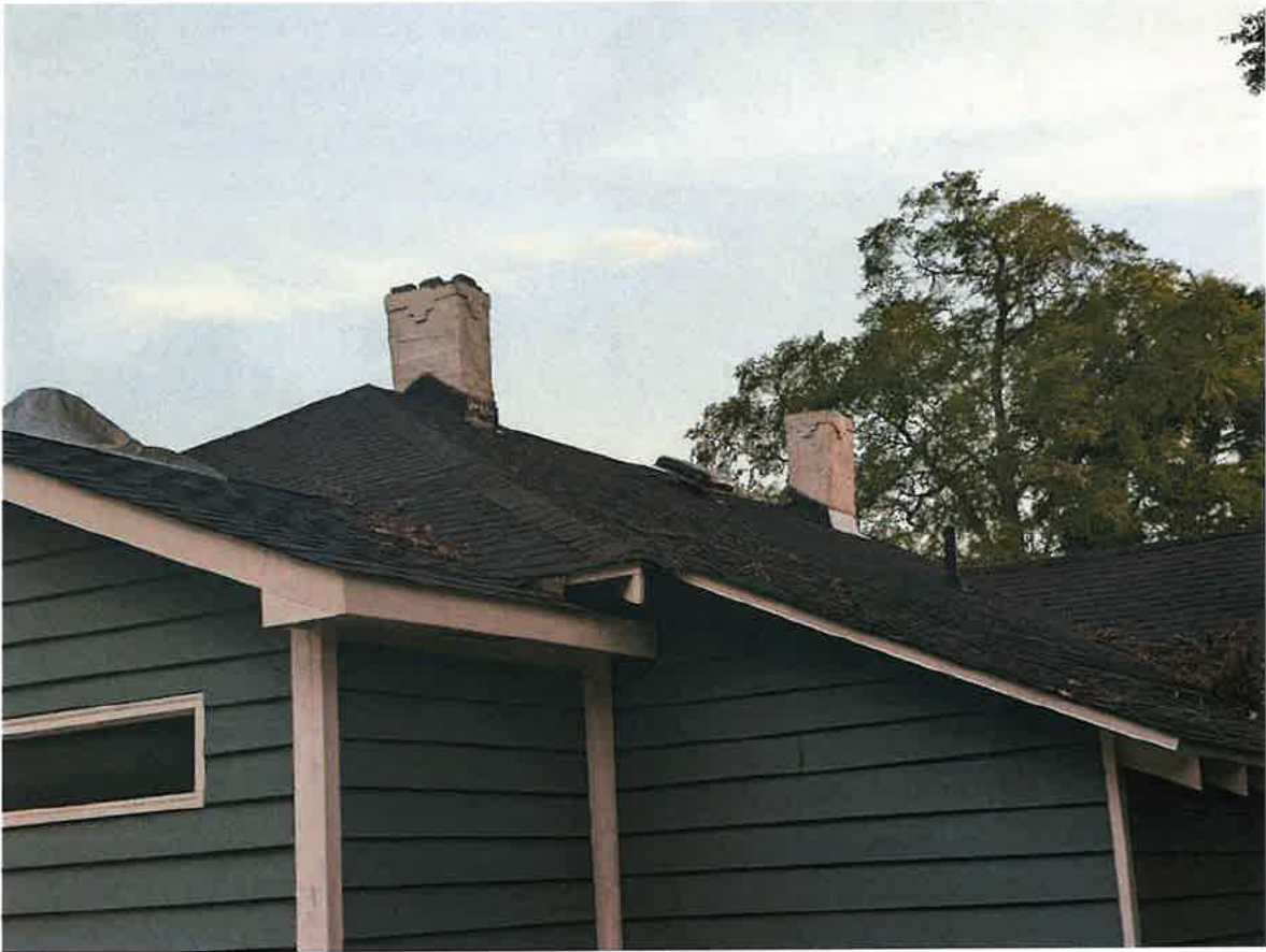
Subject property 902 Washington Street Rear Left
