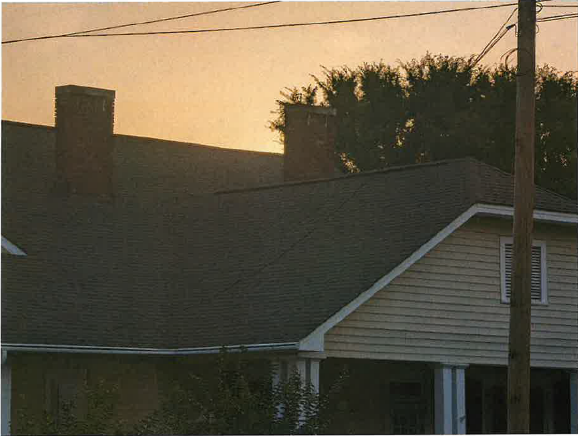
Roof of 907 Washington Street with ridge vent
