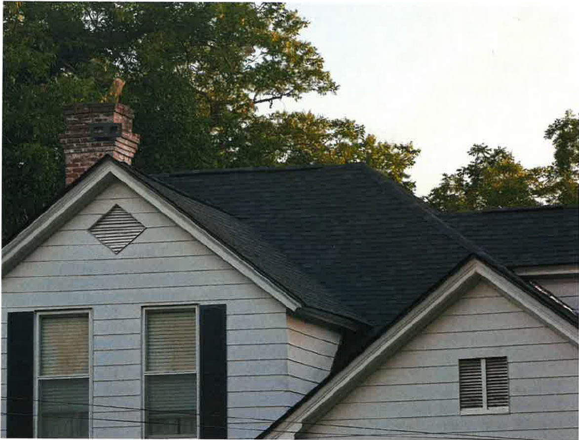
Roof of 901 Washington Street with ridge vent
